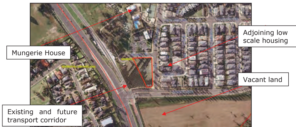
Figure 7 Lavender Field Site
